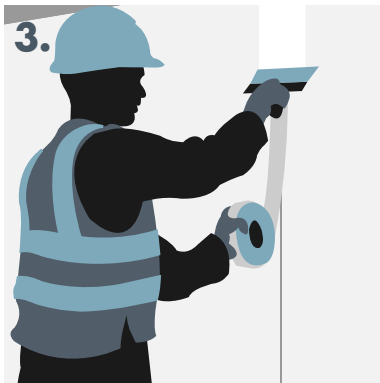
3. Embedding Knauf Aquapanel Exterior Joint Tape.
